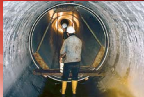
Ideal pipe for rehabilitating corroded sewers
